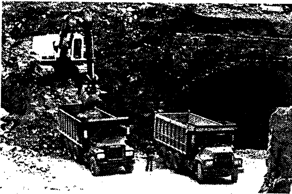
FIGURE 12. — Old railroad tunnel exposed during excavation at Steel Plaza Station.
